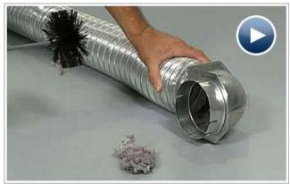
Lint, that seemingly harmless fluff that you pick off your clothes, causes thousands of residential fires in the U.S. each year. Dryer venting can become clogged with the stuff, causing a dangerous buildup of heat and, too often, a fire. Here's how to prevent dryer fires:
